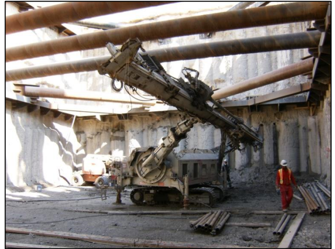
PG-115 in drilling position
